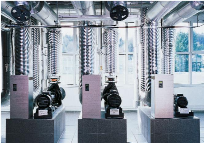
Boiler flow rates controlled by variable speed pumps
