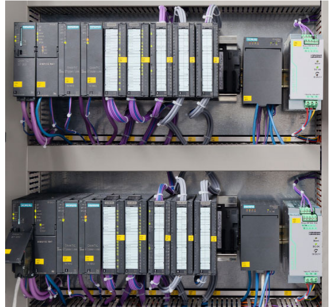
Highest safety provided by 100% redundancy of burner control systems
